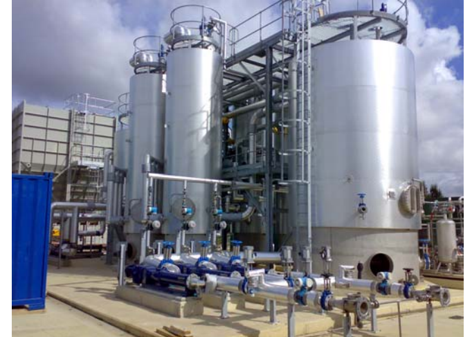
Typical Thermal Hydrolysis Plant
